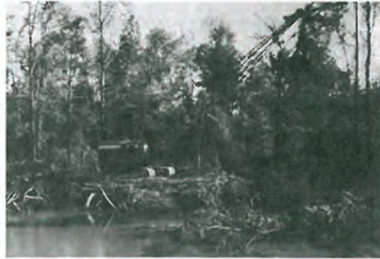
Figure 17. Dragline being used to remove compacted debris and sediment at major blockage (Condition Four).
