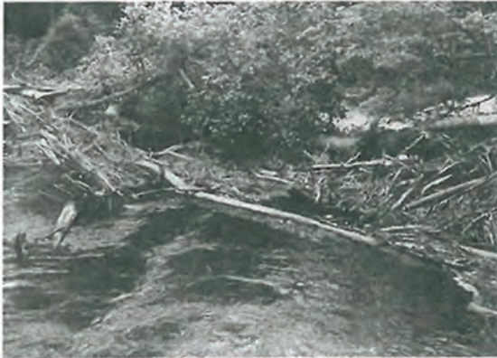
Figure 5. Log crossways of stream channel, trapping additional debris and restricting flow. Flow problems are likely to increase in the near future. Such accumulations may be removed.
