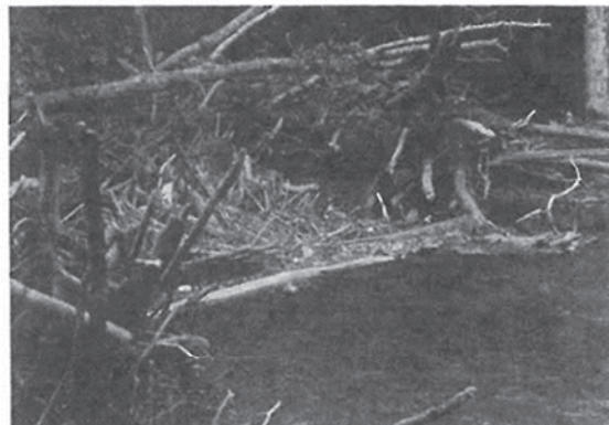
Figure 3. Debris accumulation obstructing flow and is likely to cause additional problems. Such accumulations may be removed.
